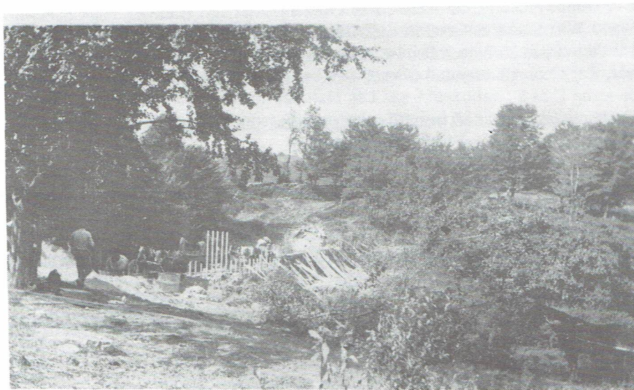
Work being done on the original Muskoday dam, 1921.
